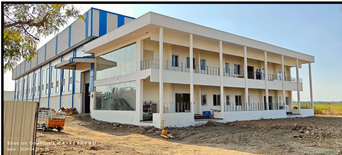
Propel – Drive Building View (Actual Images – View 1)
