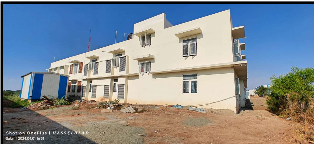
Propel – Hostel Building (Actual Images – View 3)
