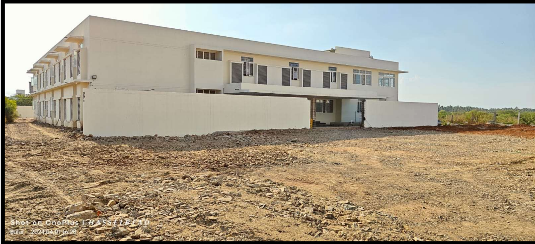
Propel – Hostel Building (Actual Images – View 1)
