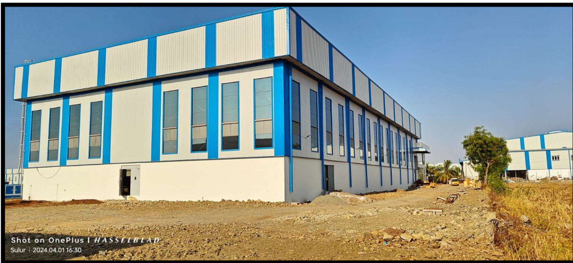
Propel – Drive Building (Actual Images – View 3)
