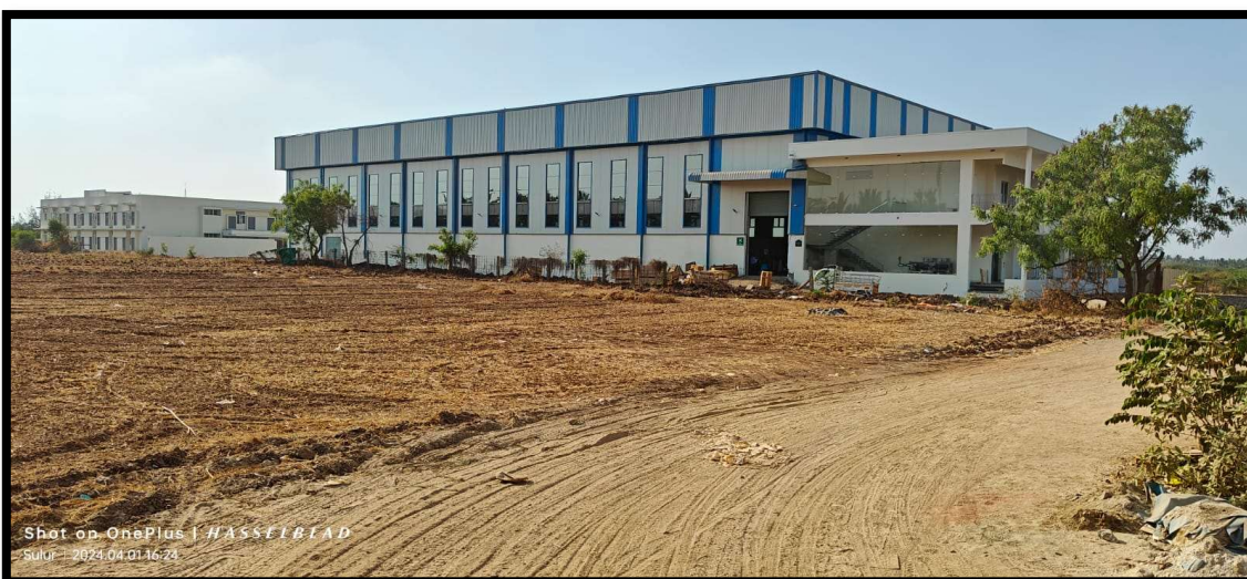
Propel – Drive Building (Actual Images – View 4)
